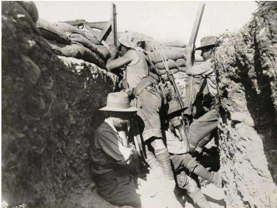
The Periscope Rifle saved many soldiers' lives as it allowed them to see the enemy without showing themselves over the parapet.
